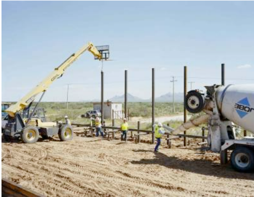
David Taylor, Pedestrian Fence Construction, NM, 2007
